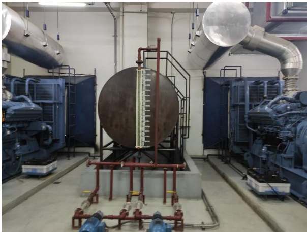
AC Electric Generator Sets
