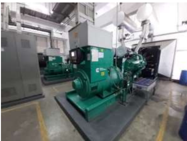
Stand-by AC Electric Generating
