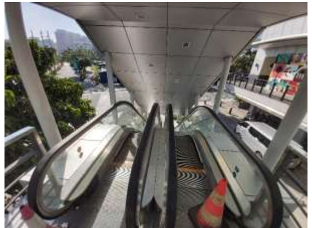
Escalator adjacent to commercial spaces
