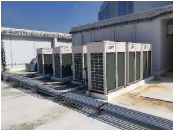
Air Conditioning Units
