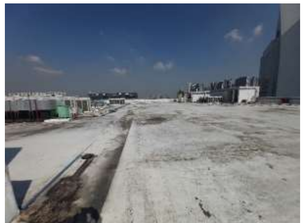
Roof Deck Area
