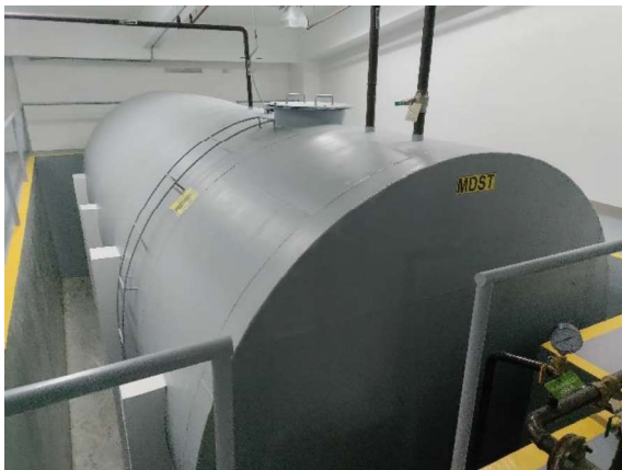
Diesel Fuel Tank
