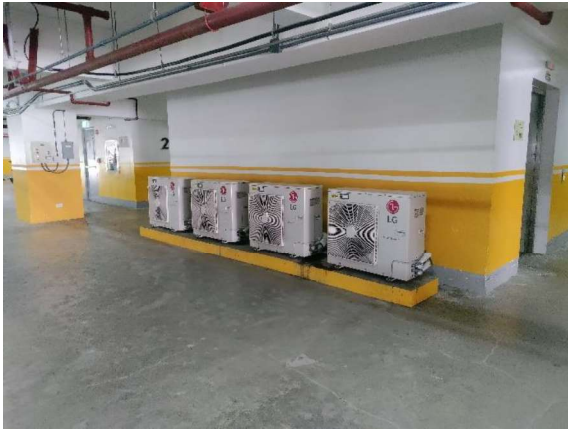
Air-cooled Condensing Units
