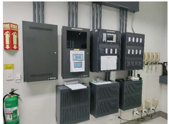
Fire Detection and Alarm Control Panel
