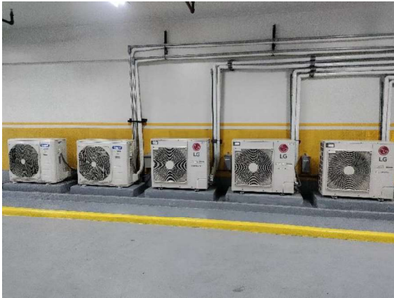
Air-cooled Condensing Units
