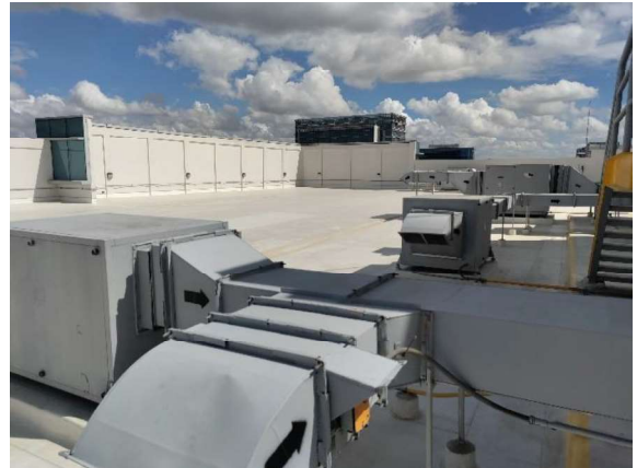
Air Ventilation and Exhaust System
