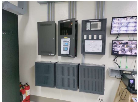
Fire Detection and Alarm Control Panel
