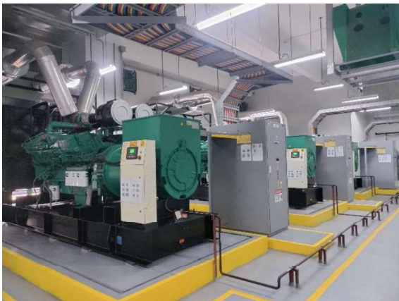
AC Electric Generating Sets
