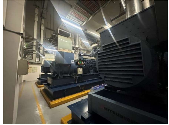
AC Electric Generator Sets
