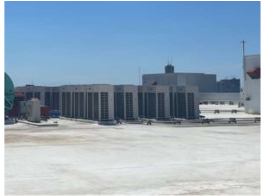
VRF Airconditioning Units
