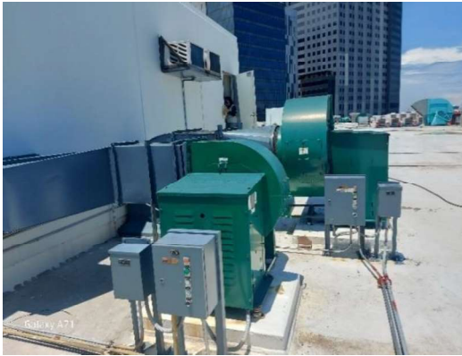
Supply and Exhaust Fans
