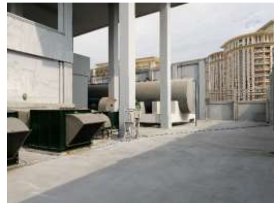
Overhead Water Tanks
