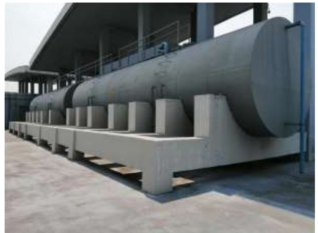
Overhead Water Tanks
