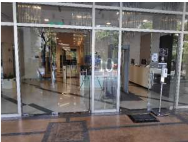
Main Entrance of Lobby 10
