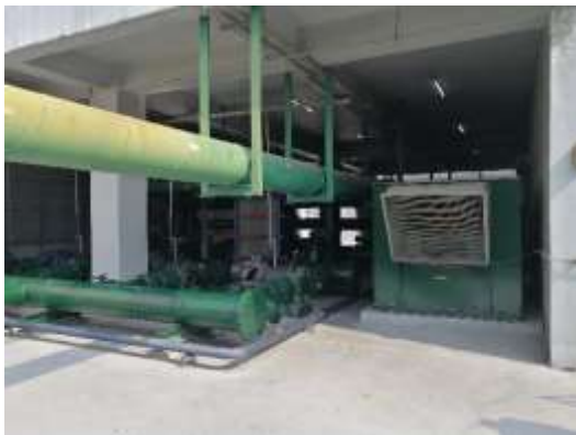
Air Conditioning Units / Cooling Tower
