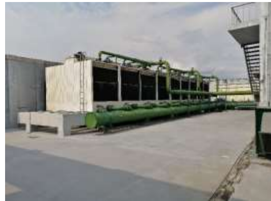
Air Conditioning Units / Cooling Tower
